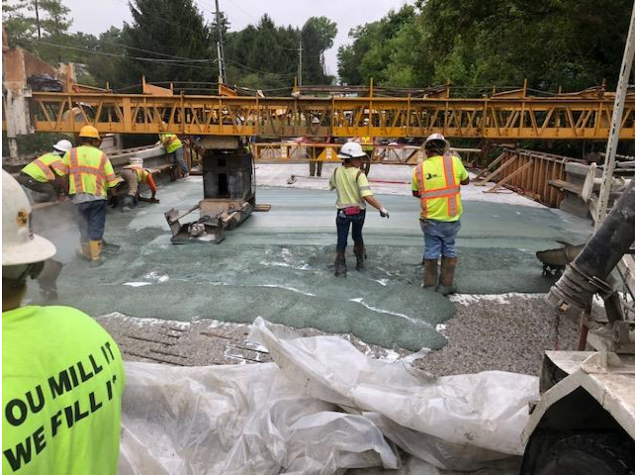
PCC latex overlay work – looking west on 116 th Street
