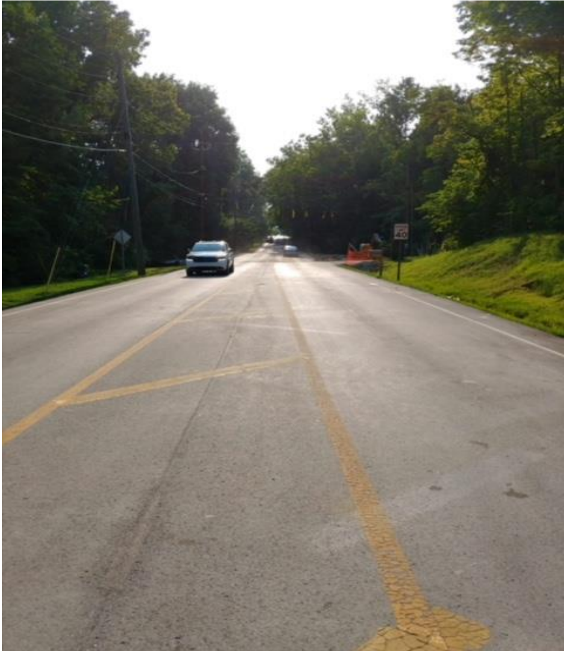
ROADWAY OPEN at Culvert #36 – looking west along 116 th Street.
