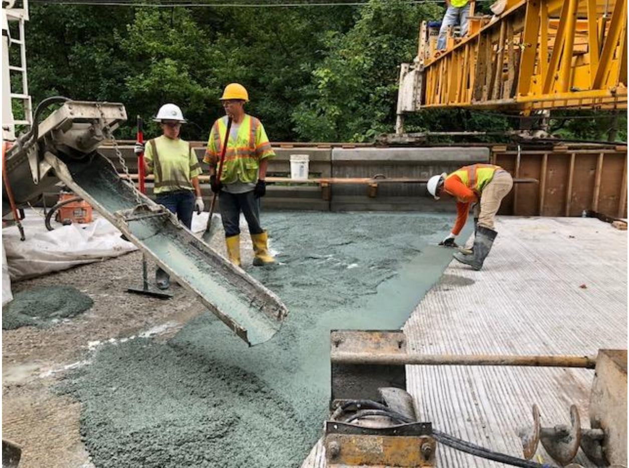
PCC latex overlay work – looking south on 116 th Street.
