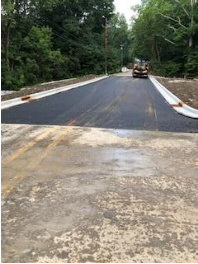
HMA Paving – looking west along 116 th Street – Culvert #36
