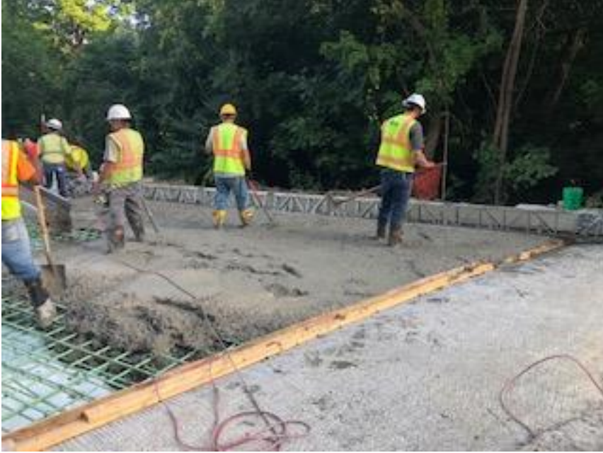
Pouring PCC approach slab – looking north from 116 th Street
