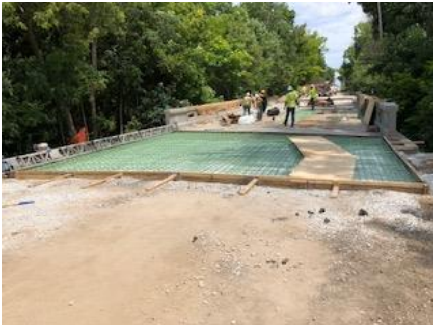
PCC approach slab form work – looking east on 116 th Street
