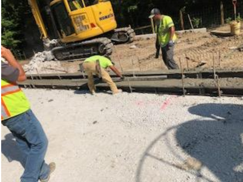
PCC Curb placement @ Culvert #36 – looking north from 116 th Street
